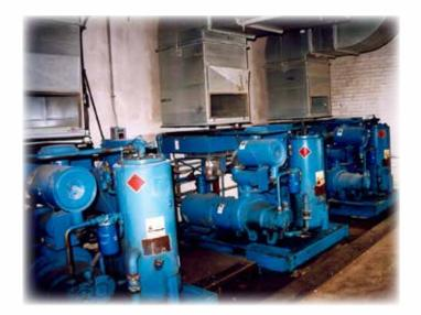
the previous commercial grade oil. Later, the decision was made to extend oil, filter and separator changes out to 3,000 hours vs. the previous 2,000 hours.
